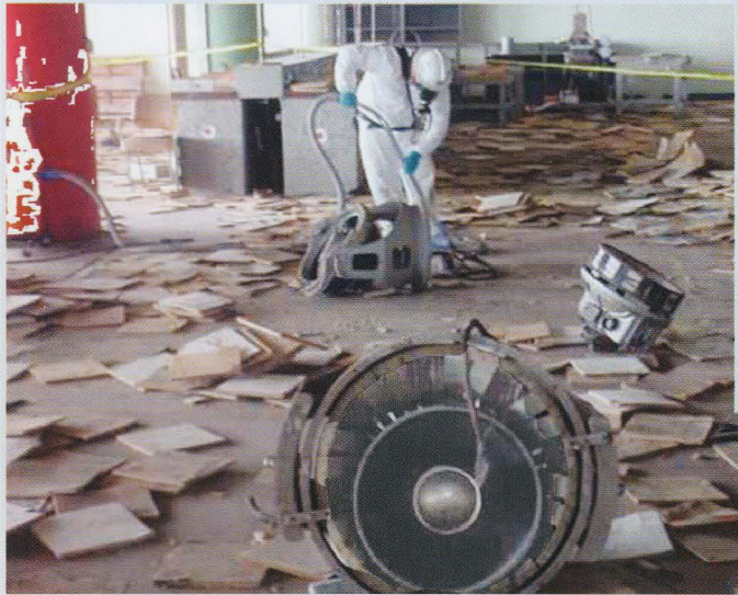
Below: A High Efficiency Particulate Air (HEPA) filtration system is used to remediate suspected asbestos contamination in Building 235.
