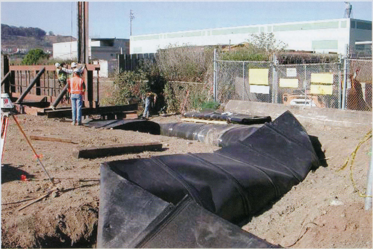
Installation of the barrier wall
