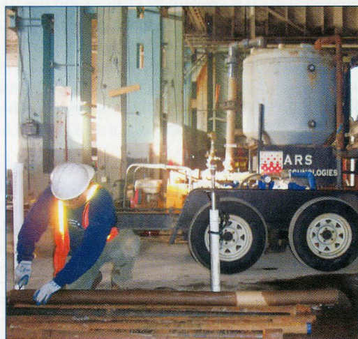
ZVI slurry is mixed in the mobile tank and injected in TCE-contaminated areas.
